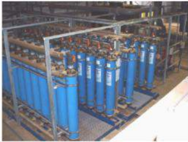
Figure 1: HYDRAcap Installation at Seedy Mill WTW
